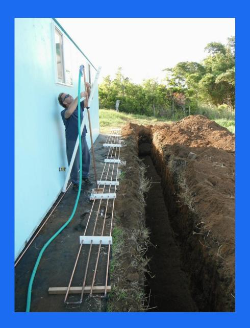
Geothermal cooling ditch with copper cooling coil
